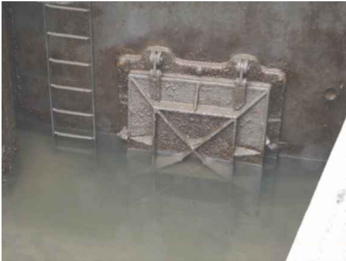
Figure 3.8. The outer flap in the structure shown in Figure 3.4. Note that the flap is being prevented from complete closure by two plastic bottles jammed in the gap, one on each side. While this serendipitous situation would allow some landward flow and passage of elvers were this a single flap, the presence of a second flap a couple of metres behind this one, prevents this.
