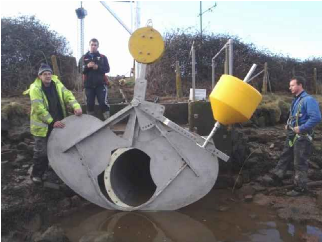
Figure 4.4. Williams/Stoneman SRT gate during installation on the Axe Estuary, Devon
