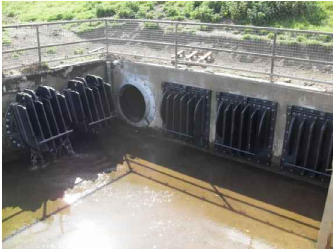
Figure 3.11. A range of lightweight HDPE tidal flaps, supplied by Aquatic Control Equipment (ACE) Ltd. Photograph courtesy of ACE.
