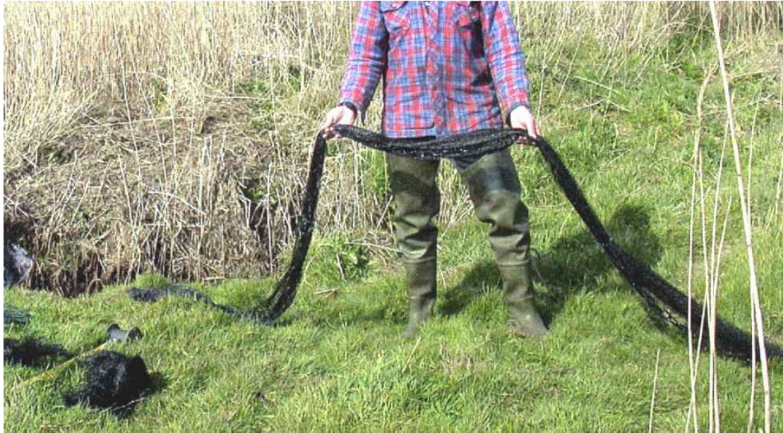
Figure 3.21. Chain wrapped in garden mesh prior to installation at Lodmoor.
