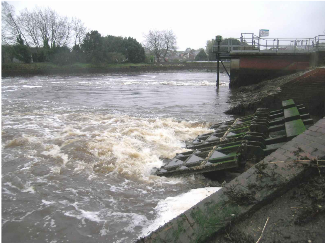
Figure 3.13. The counter-weighted flaps on the Lymington River, fully open during a spate. The flow of water in the middle distance is from the tidal gates shown in Figure 3.2.
