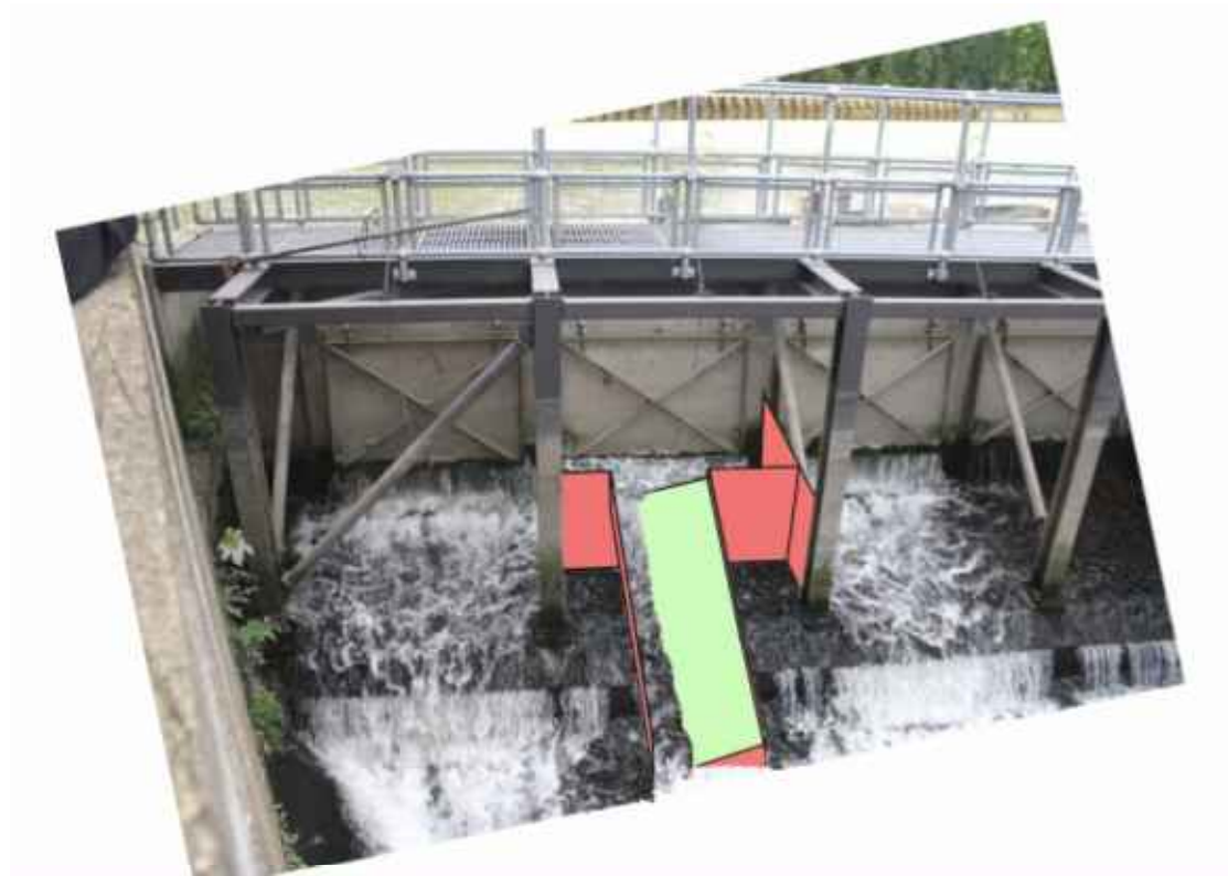
Figure 3.25. Schematic diagram of a proposed gravity-fed elver pass at a tidal flap at Three Mills Weir at the tidal limit of the River Lea in London. This option is made possible by the carefully-maintained head in the navigation channel upstream, and the availability of alternative routes for flow so that the reduction in flood flow capacity is of no consequence.
