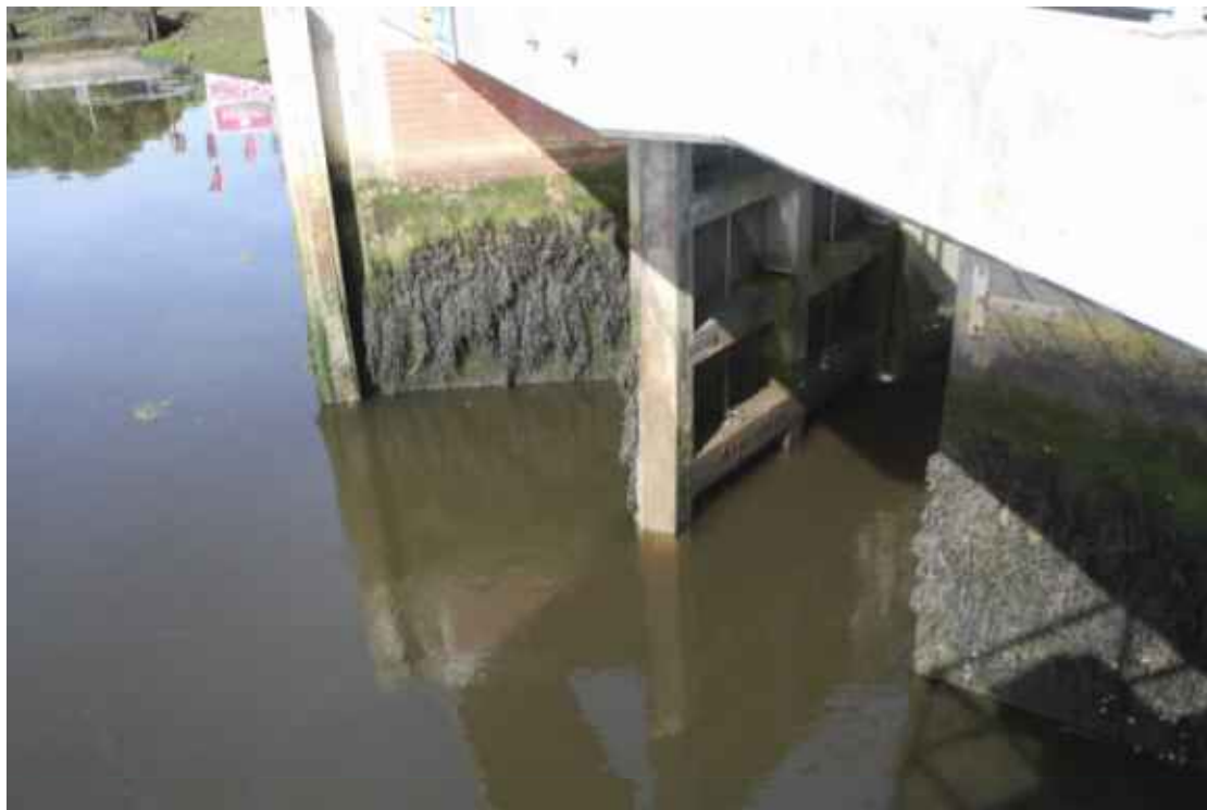
Figure 3.3. Tidal doors on the estuary of the Lymington River in Hampshire, in an open position. The tide has started to flood, and there was noticeable landward flow (towards the right of the picture) through the structure when this picture was taken. A few minutes later as the landward flow increased, the doors slammed shut.
