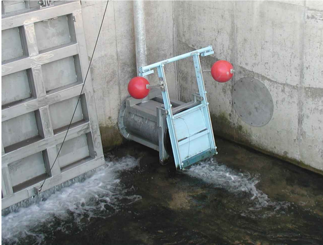
Figure 4.3. Waterman SRT gate installed alongside a much larger tidal flap at Cone Pill. The tendency for the gate to remain open can be adjusted by swinging the floats forwards or backwards. The gate closes when the tide level rises to lift the floats. The tide level at which the gate closes can be adjusted by raising or lowering the floats. Soon after installation the floats were raised on long extension arms to keep the gate open for longer as this site has an extreme tidal range.
