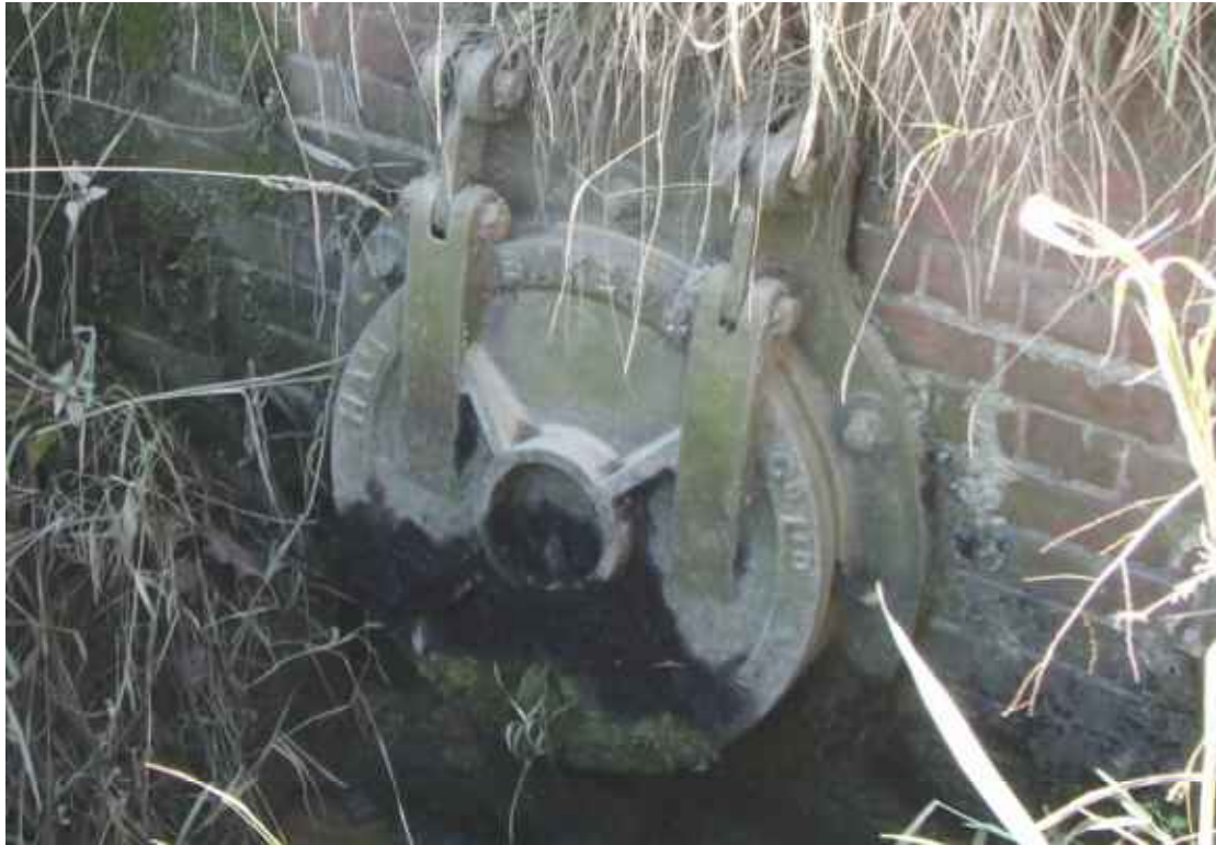
Figure 3.10. A pegged tidal flap ; note the piece of wood at the 3 o'clock position holding the flap ajar.
