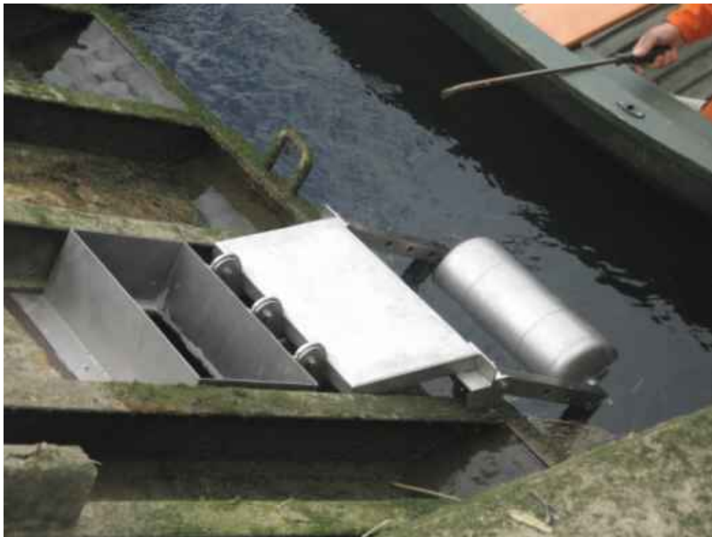
Figure 3.17. Bottom-hinged cat flap in tidal flap on the River Stiffkey in an open position. The timing of closure can be adjusted by altering the position of the float. Photograph with permission of Ros Wright, Environment Agency.
