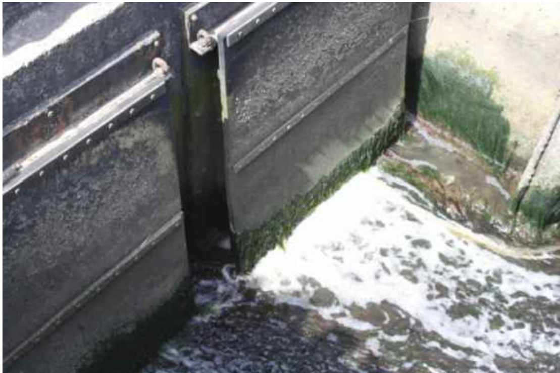
Figure 3.22. Chain wrapped in garden mesh laid through tidal flap at Lodmoor. The chain, covered in algal growth, is visible on the far side of the flow.
