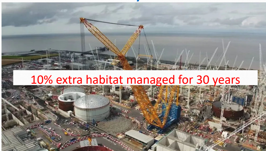
Hinkley nuclear power station
